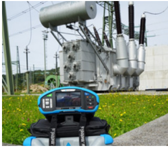
INDUSTRIAL TESTING Low Voltage Systems.
